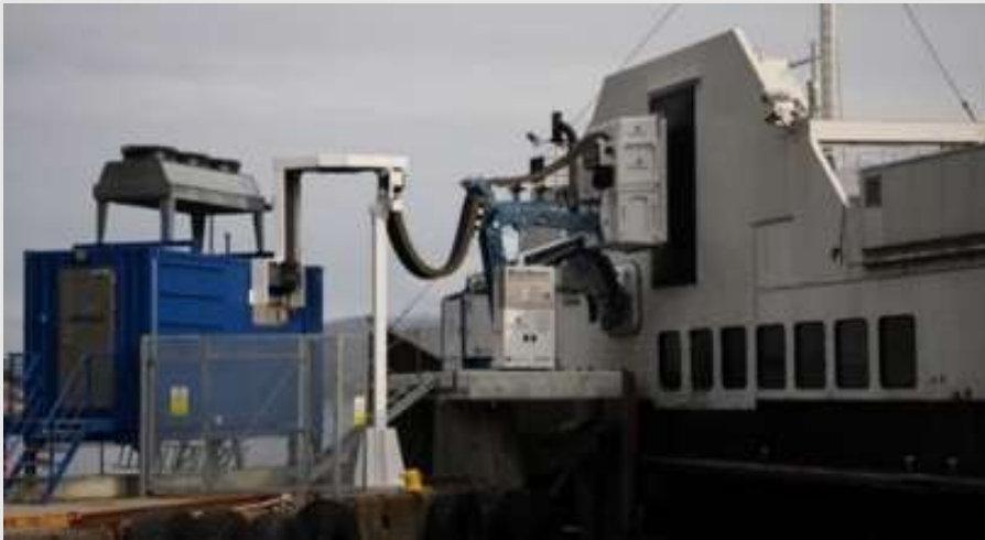
Inductive and plug charging solutions developed and tested onboard Folgefonn, Combined with vacuum mooring
